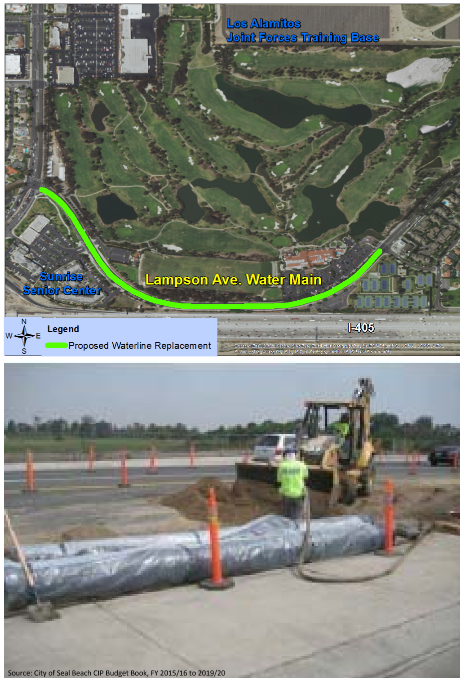
Figure 9. Lampson Avenue Water Main Project Location
